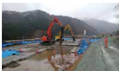
Reinforcement work on the Yatani Mine Tailings Dam No. 1.
