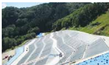
Contamination containment work at Komagi Mine: membrane section waterproofing
