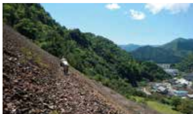
Tailings dam management (Ikuno Mine)
