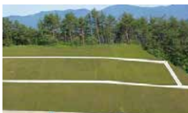
Contamination containment work at Komagi Mine: chipcrete section
