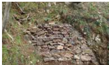
Mine drift & mine mouth management (Sado Mine)
