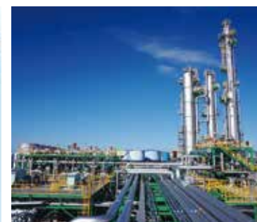
CO 2 recovery plant (courtesy of Japan CCS Co., Ltd.)
