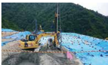
Reinforcement work on the Washiainori Mine Ketakura Tailings Dam.
