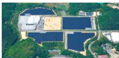
Yabuki Solar Power Plant
