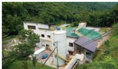
Mine wastewater treatment management (Teine Mine)
