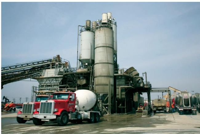
North American Ready-Mixed Concrete Plant (RRM)
