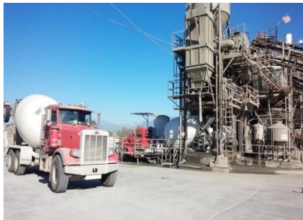
RRM Ready-Mixed Concrete Plant
