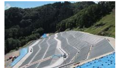
Contamination containment work at Komagi Mine: membrane section waterproofing
