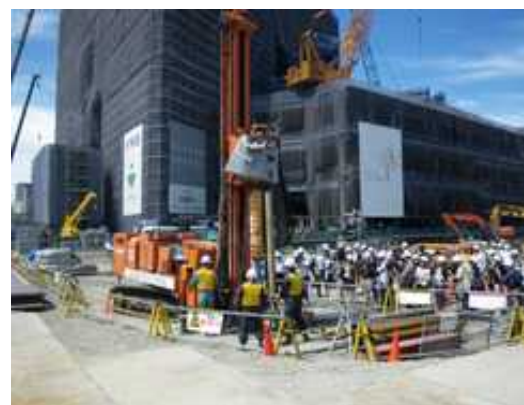
Construction of in-ground heat exchanger well at Tokyo Sky Tree
