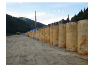
Reinforcement work by soil stabilization at the Yatani Mine Tailings Dam
