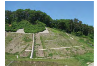
Contamination containment work by slope seeding called Chip-creteat the Komagi Mine
