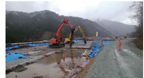
Reinforcement work on the Yotani Mine Tailings Dam No.1
