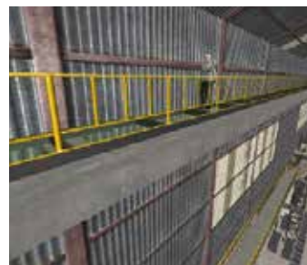
Falling accidents (stepping through the floor)
