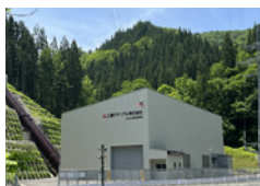
Tohoku Power Service Station (Komatagawa New Power Plant)
