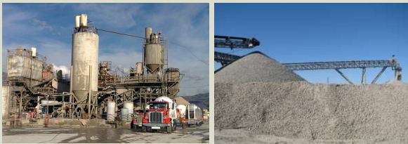
Ready-mixed concrete plant
