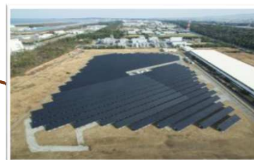
Mega solar: Fukui Photovoltaic Power Plant, Fukui, Fukui Pref.
