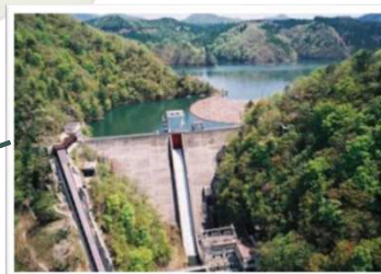
Hydroelectric: Moriyoshi Dam, Akita Pref. Komatagawa No.4 Hydroelectric Power Plant
