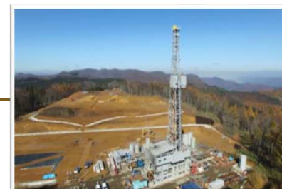
Geothermal power: Yuzawa, Akita Pref. (Wasabizawa, under construction)
